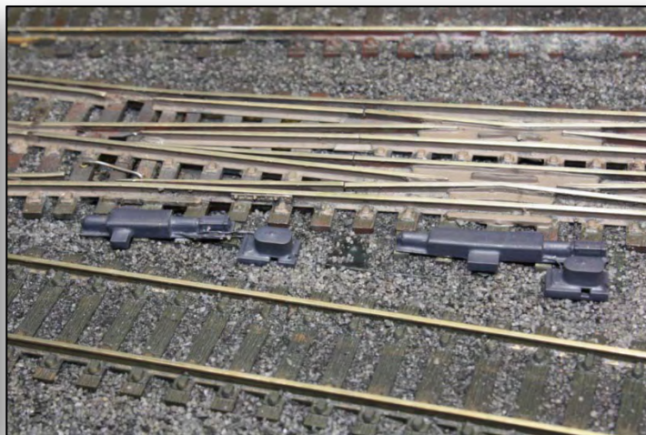
The switch machine on the left has a non-standard CP valve position due to tight clearances.
