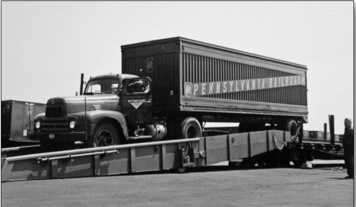
A 30' LCL van being test loaded on F30D TrucTrain Flat Car. Note the heavy corner posts, bottom sill, and scuff bands designed to protect the trailer body in the tight confines of eastern cities. (Curt LaRue collection)
