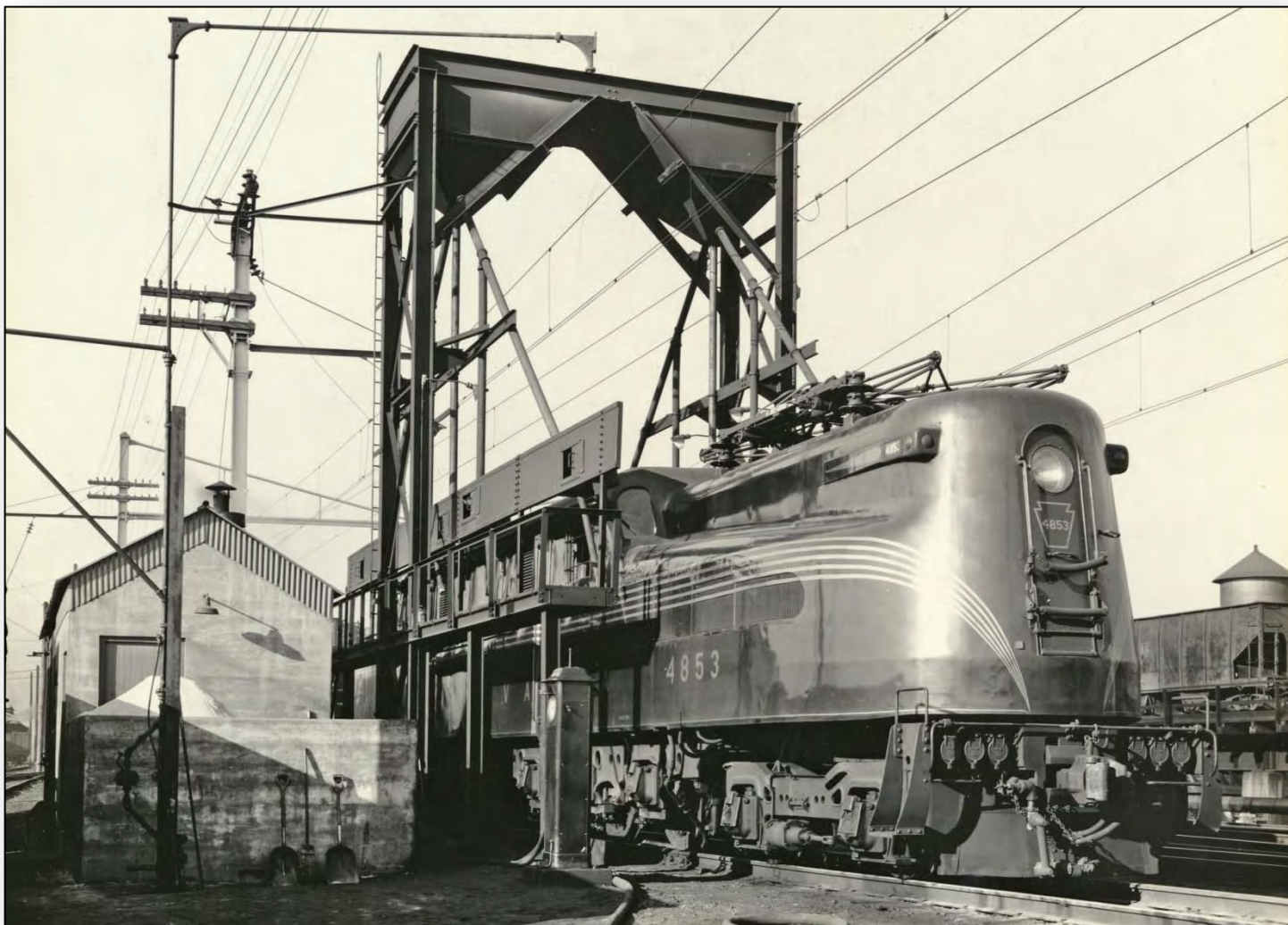
Prototype: GG1 #4863 in the Sanding Tower at Harrisburg. (Collection of Andy Hart)
